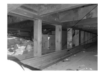
EXISTING WOOD JOISTS, KNEE WALL FRAMING AND STAGE FLOOR CONSTRUCTION TO BE REMOVED IN ITS ENTIRETY
